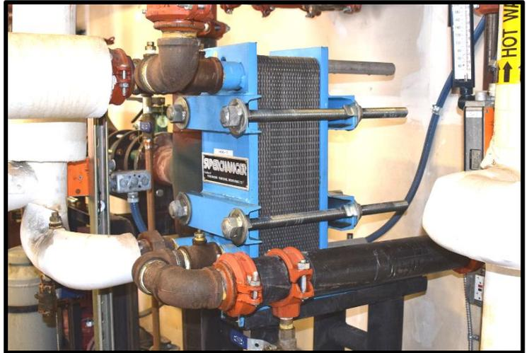
I did charge the building for my time but the end result is a significant savings over the other contractors cost. An extra advantage in doing it "in-house" is the plates themselves are factory re-fabricated units and essentially are brand new, a substantial improvement over scraping off the old gaskets by hand with a chisel and gluing new ones back on in the field. Also, the old plates can be sent to the factory to be refurbished to a new condition for the next servicing at a much reduced cost.
