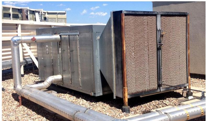
Figure 1 -- Rooftop Make-Up Air Unit (MAU). Air is drawn from the square structures on the right. It is filtered then cooled or heated and delivered to the hallways on all floors through ductwork in the ceilings.
